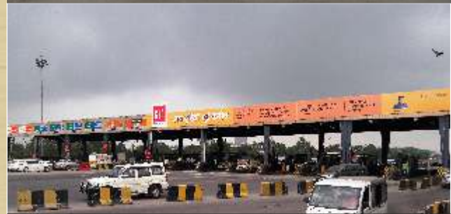
National Highway 8 : approx. 1.4 kms. Dwarka Expressway : approx. 350 meters
